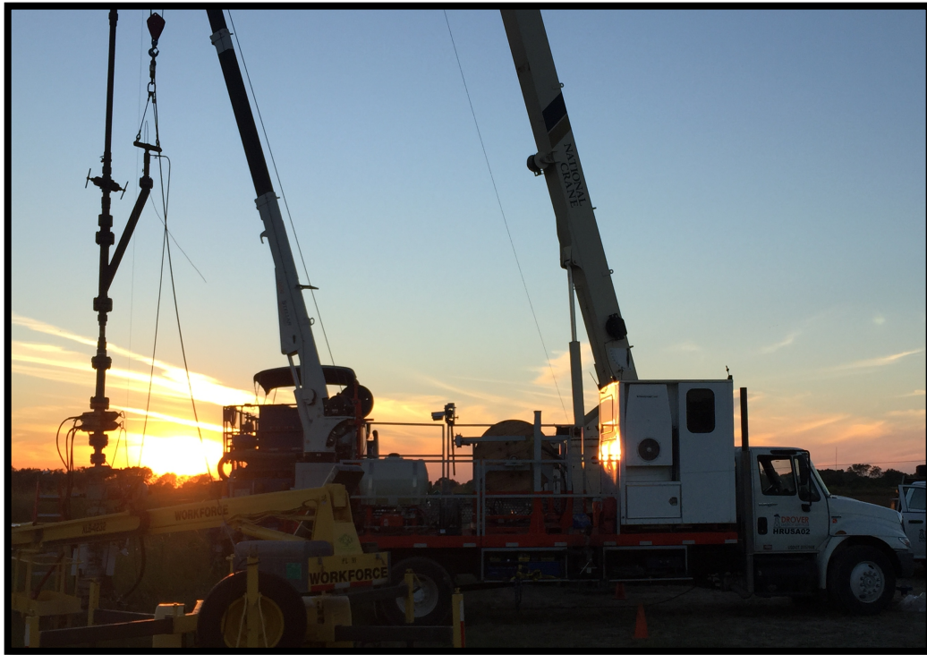
Figure 3-- Y-Body Rig Up Stroking Tubing Out of Working Packoff, with BOP assembly.
